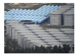
Fig. 1. Tanks in the Fukushima Daiichi Nuclear Plant. The tanks are used to store contaminated water.
