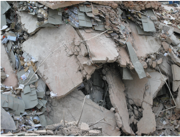
Fig. 6. Mixture of debris. It is composed of ferro-concrete, concrete and bricks of walls, as well as interjacent shelves and historical documents. As shown, there are hardly no voids, where possible victims could have survived [1].
