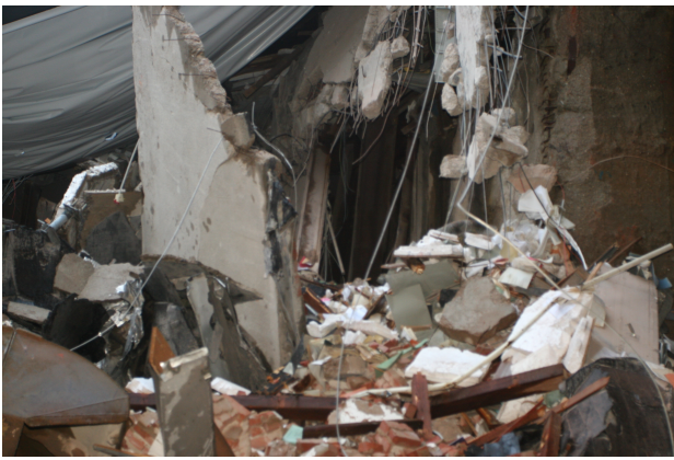
Fig. 12. Detail view of the scene in Fig. 10. What can be seen are so called widow-makers endangering the operators [1].
