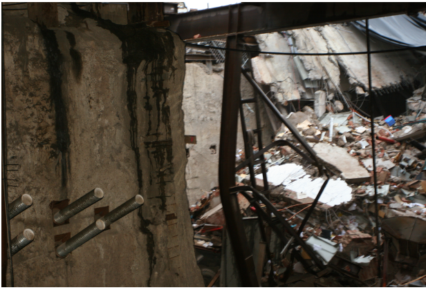
Fig. 11. Bent H-carrier next to the operating area of the Active Scope Camera [1].
