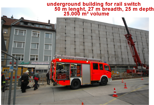
Fig. 2. The rail-switch station and the subway tracks are located below the horizontal concrete paving slabs in front. This picture has been taken four weeks before the collapse [1].
