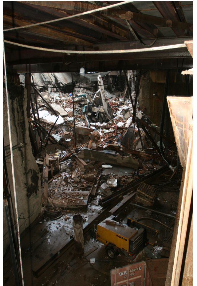
Fig. 10. Subsurface scenery. On the right-hand side the rail-switch is shown. The victims had been expected on the left side, behind the perforated slotted wall. The Active Scope Camera could have been employed in this situation, but the operating area was not safe [1].
